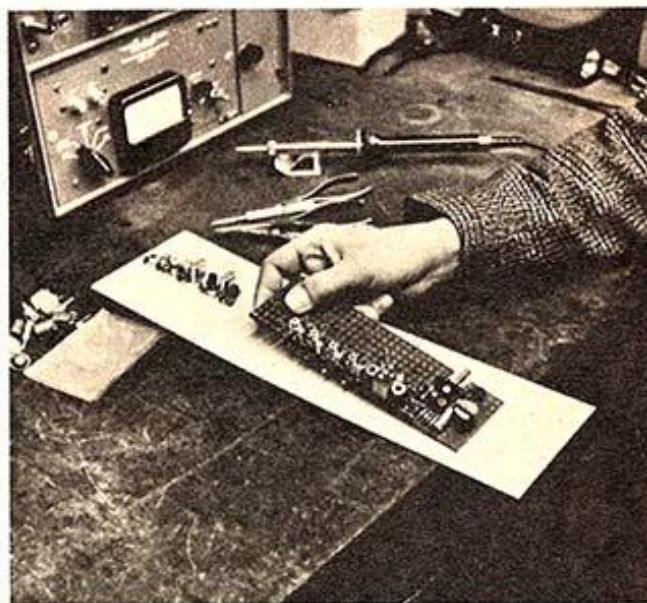
Transistorized version of transceiver is under construction; whole circuit will fit on board.
